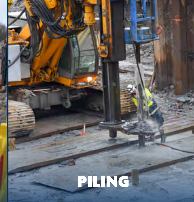
SHEET PILE DRIVING
